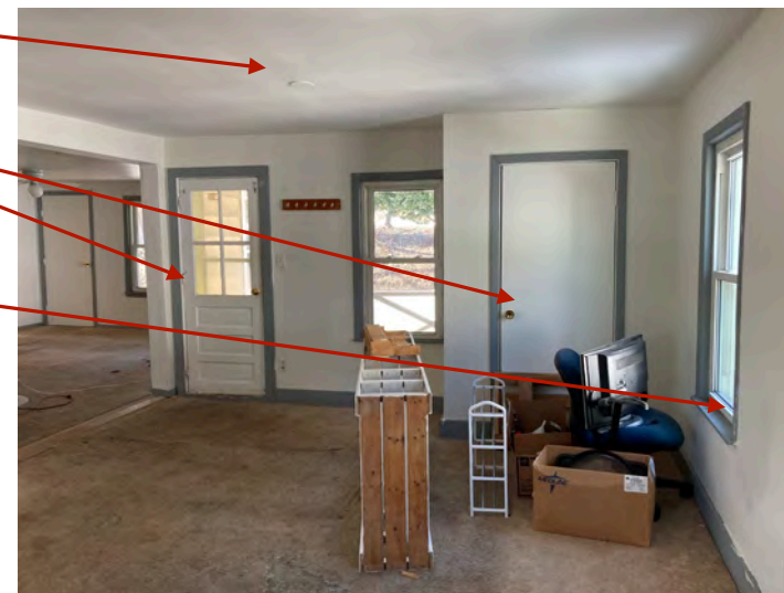
View into Existing Entry
