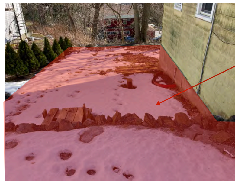
Area between the two buildings
