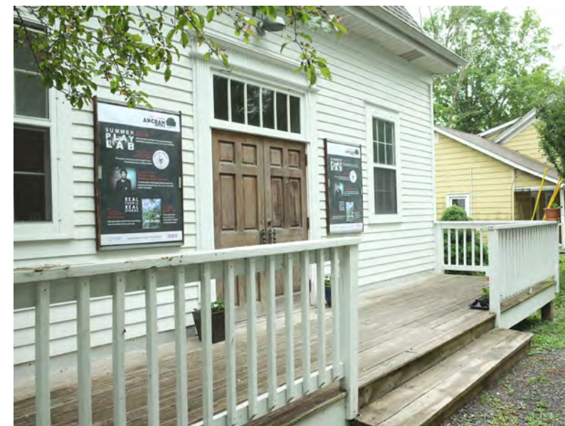
Ancram Opera House Front Entry Porch
